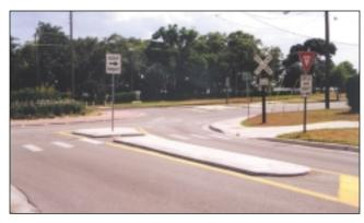
All except mini-roundabouts have raised splitter islands. These are designed to separate traffic moving in opposite directions, deflect entering traffic, and to provide opportunities for pedestrians to cross in two stages. Mini-roundabouts may have splitter islands defined only by pavement markings. *Tavares, FL*
