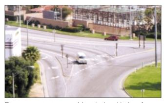
Flare on an entry to a roundabout is the widening of an approach to multiple lanes to provide additional capacity and storage at the yield line. Long Beach, CA
