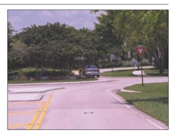
Good roundabout design requires entering vehicles to negotiate a small enough radius to slow speeds to no greater than 50 km/h (30 mph). Once within the circulatory roadway, vehicles' paths are further deflected by the central island. *West Boca Raton, FL*
